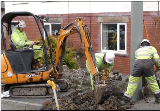
Backfilling – Excavated material is re-used to backfill around the new pole using the Bob-cat excavator.
