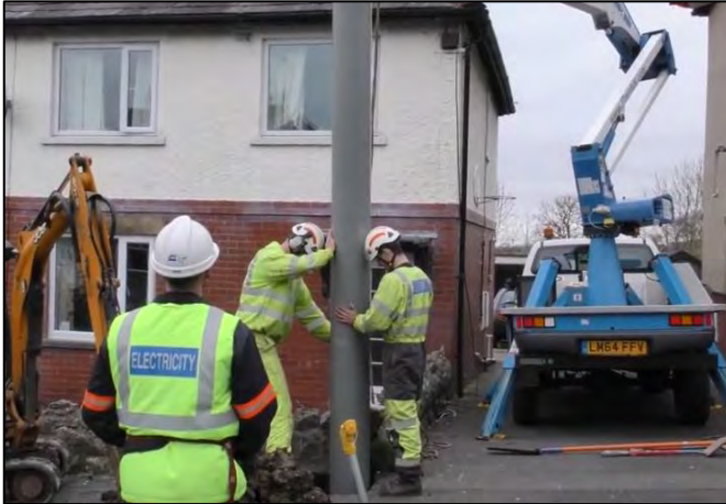
Placement of New Pole – Workers help maneuver the pole into the existing hole.
