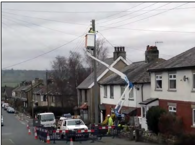
Stringing the Line – The line is replaced by a worker using the cherry picker. Any waste materials are then removed from the work area which is swept and then any fencing and warning signs are removed before moving on to the next pole.
