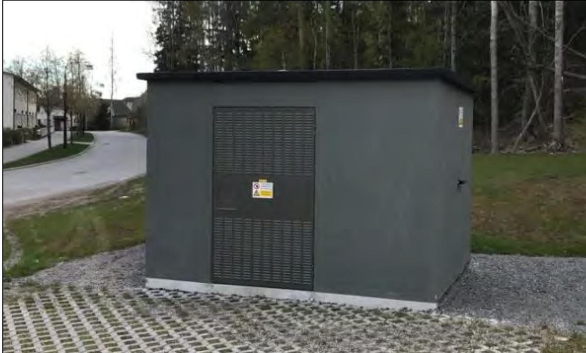
Figure 12: Pad-Mounted 'Kiosk' Transformer
