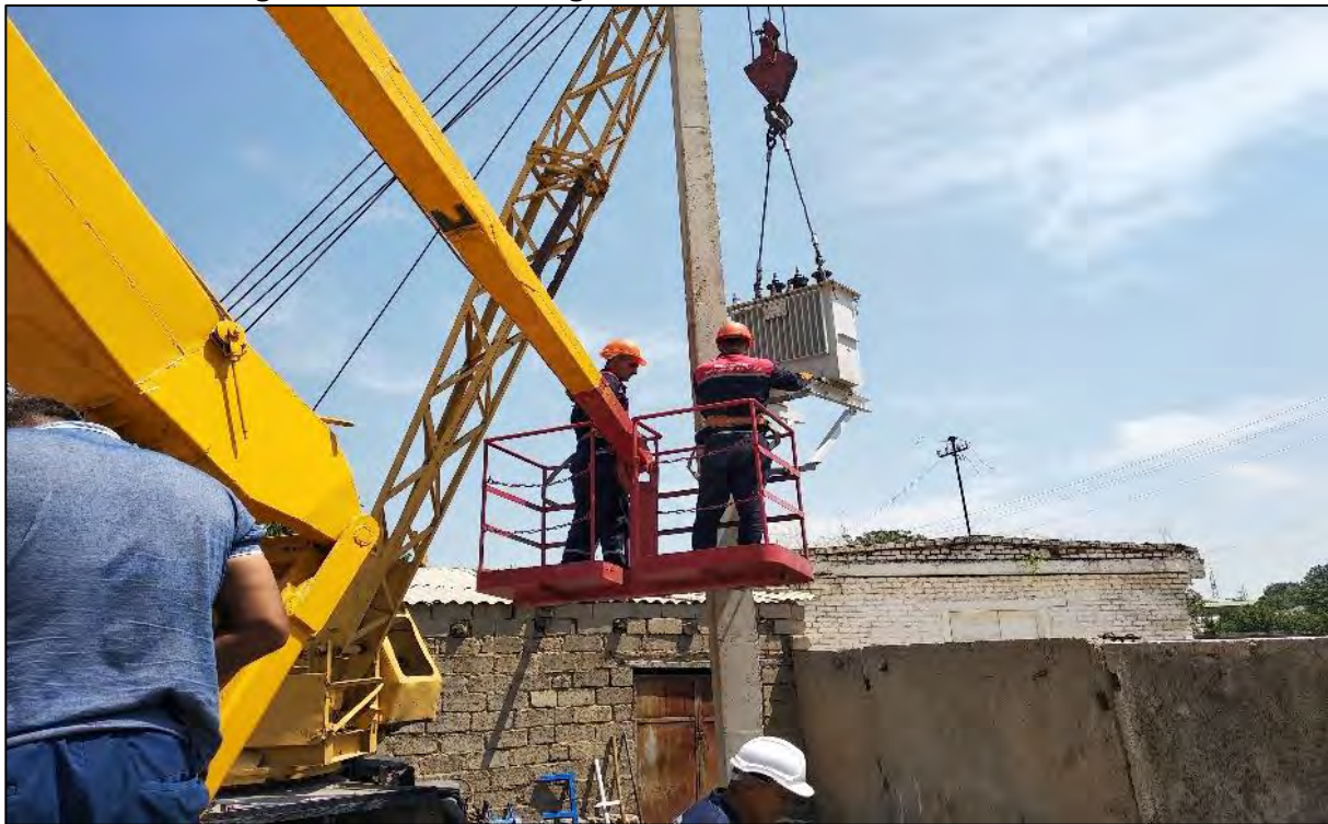
Figure 9: REN Installing a Pole Mounted Transformer, Jizzak
