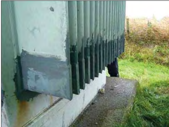
Figure 28: Fin Corrosion
