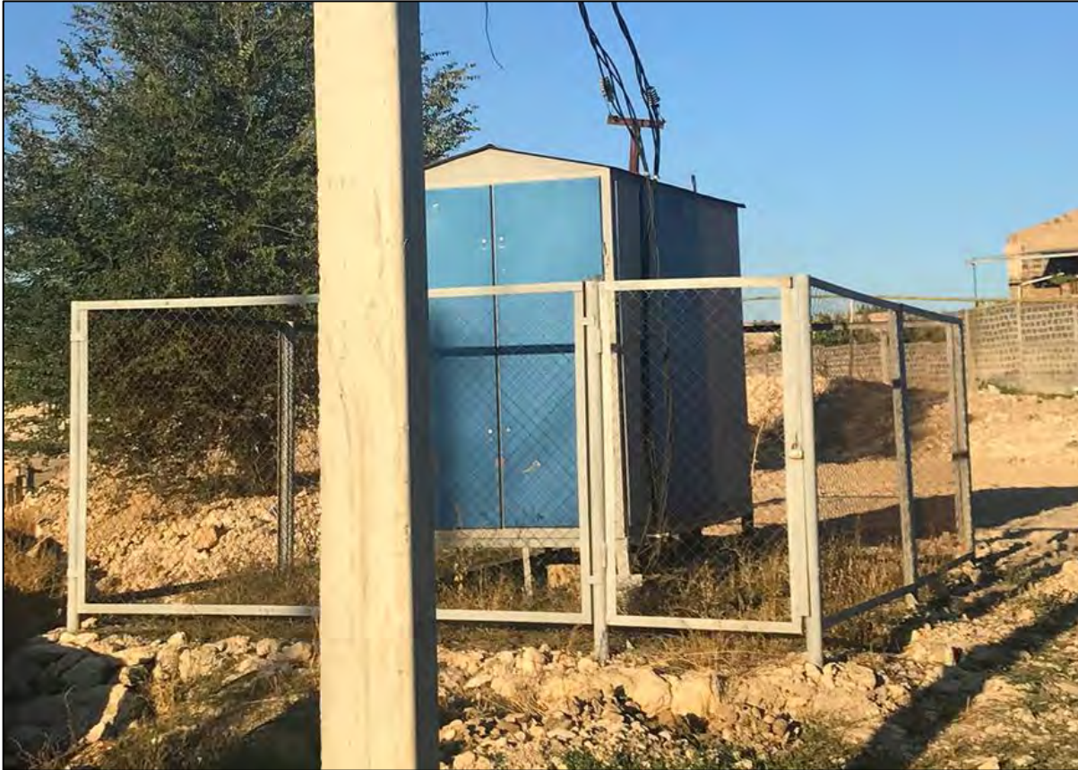
Figure 13: Pad-Mounted 'Kiosk' Transformer
